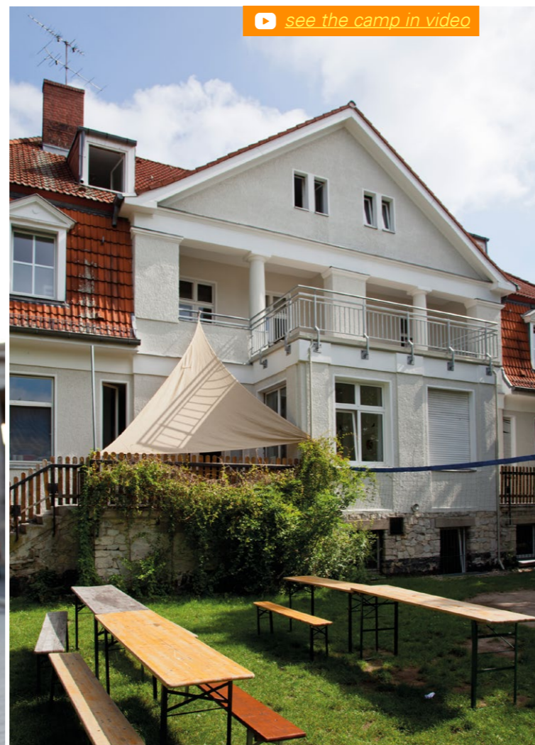
THE VILLA, CLASSROOMS ON THE GROUND FLOOR, BEDROOMS UPSTAIRS
